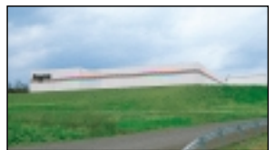
State-of-the-Art Facility, in Dallas, PA
